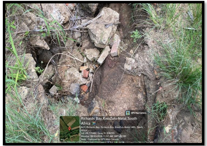
Figure 2: A drainage line was observed next to pylon 8
