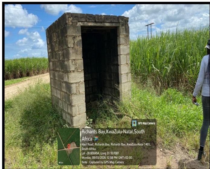
Figure 6: A fixed structure was observed on site
